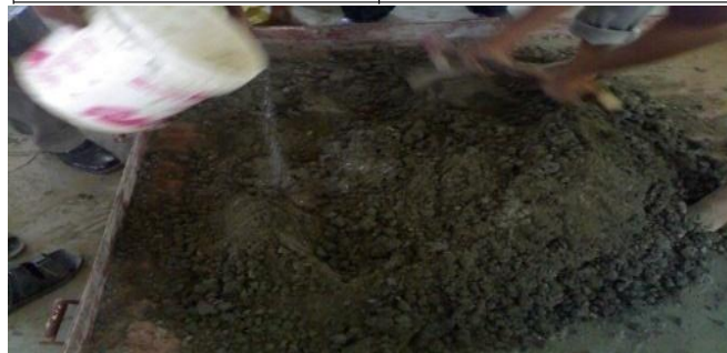
Fig. 4: Mixing of concrete
