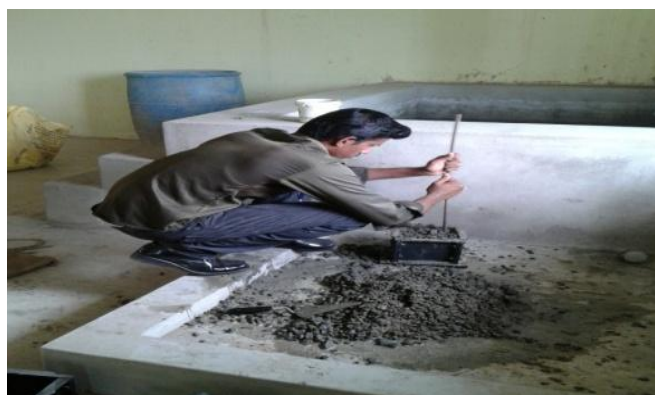
Fig. 5: Compaction of concrete
